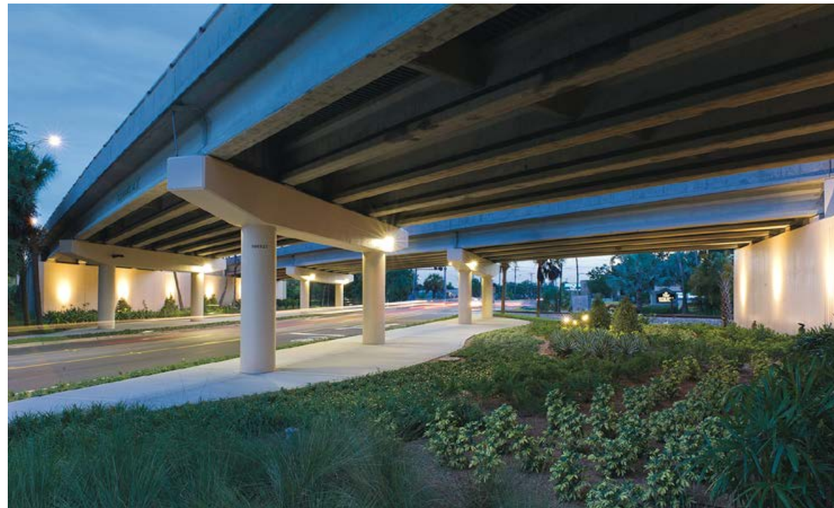
Photo courtesy of Tampa Hillsborough Expressway Authority
