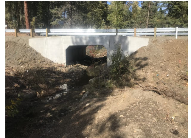
Storie Creek culvert finished in 2019
