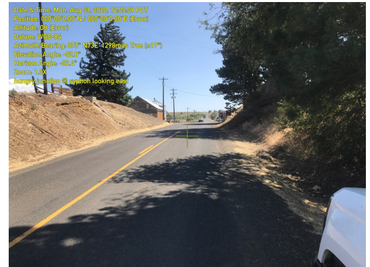
Hungry Junction Rd-Siphon
