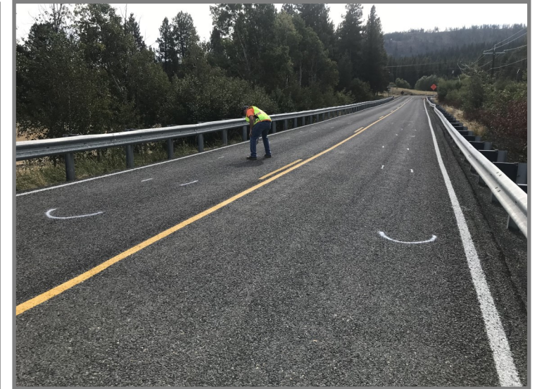
Survey work to monitor road settling
