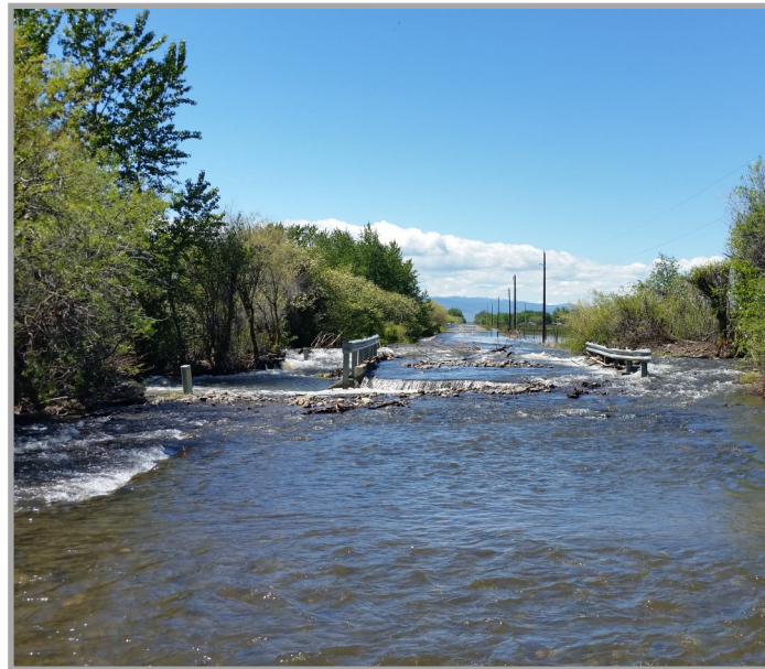
Flood event of 2017; overtopping bridge.
