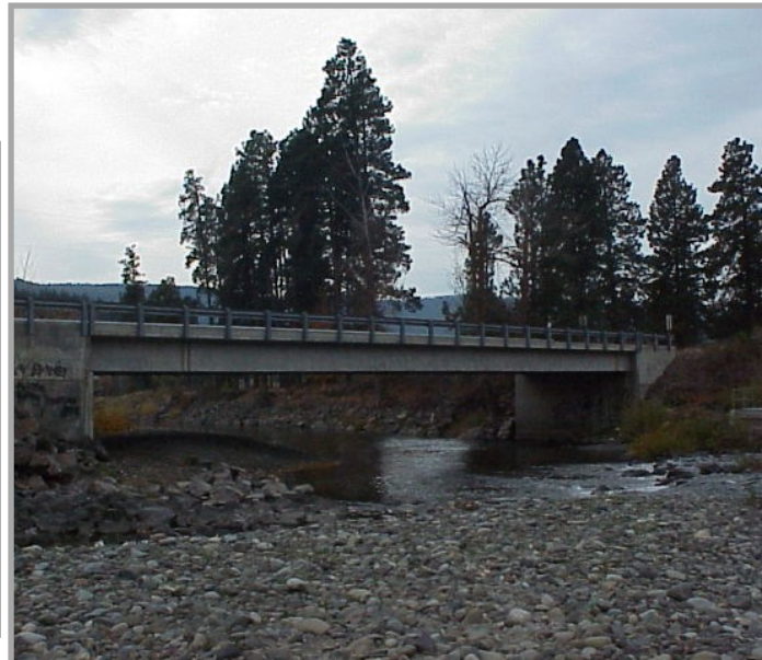
Lambert Rd Bridge over the Teanaway River
