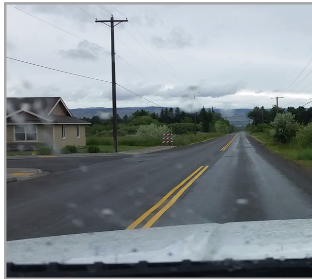
Bender Rd looking west to Reecer Creek
