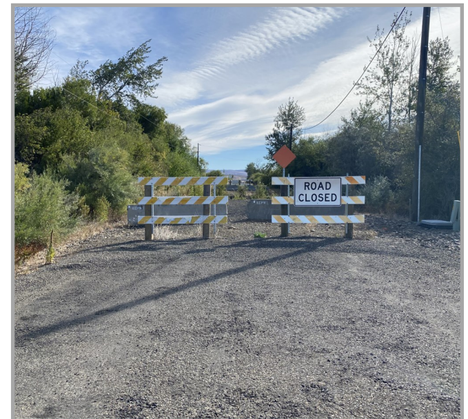
Bar 14 Rd with barricades after bridge removed.
