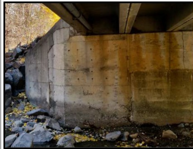
Under bridge during inspection
