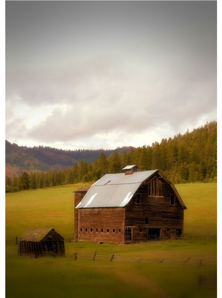
photo courtesy of Kittitas County Chamber of Commerce
