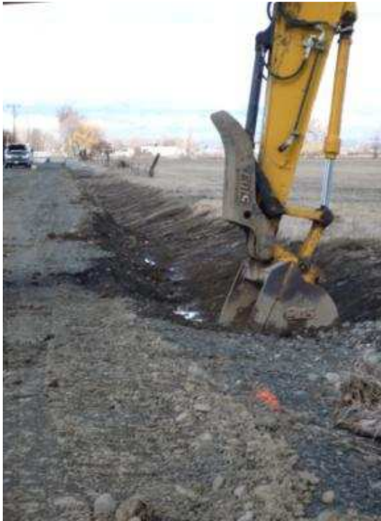
Digging Out Ditches on Ringer Loop, Preparing for Reconstruction
