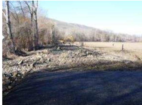
January, 2009 Flood Damage-Ringer Loop Road
