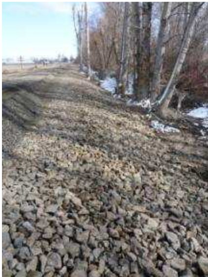
Reconstructing New Shoulders
