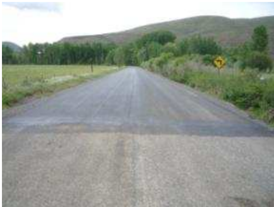
Ringer Loop Road- Paving Complete
