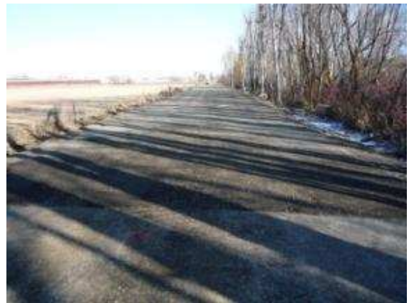
Ringer Loop Road – Reconstruction Complete - Waiting for Asphalt Prep Work
