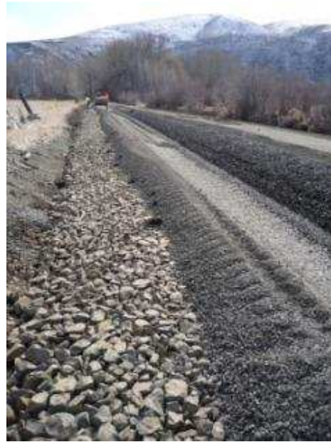
Ringer Loop Road Reconstruction
