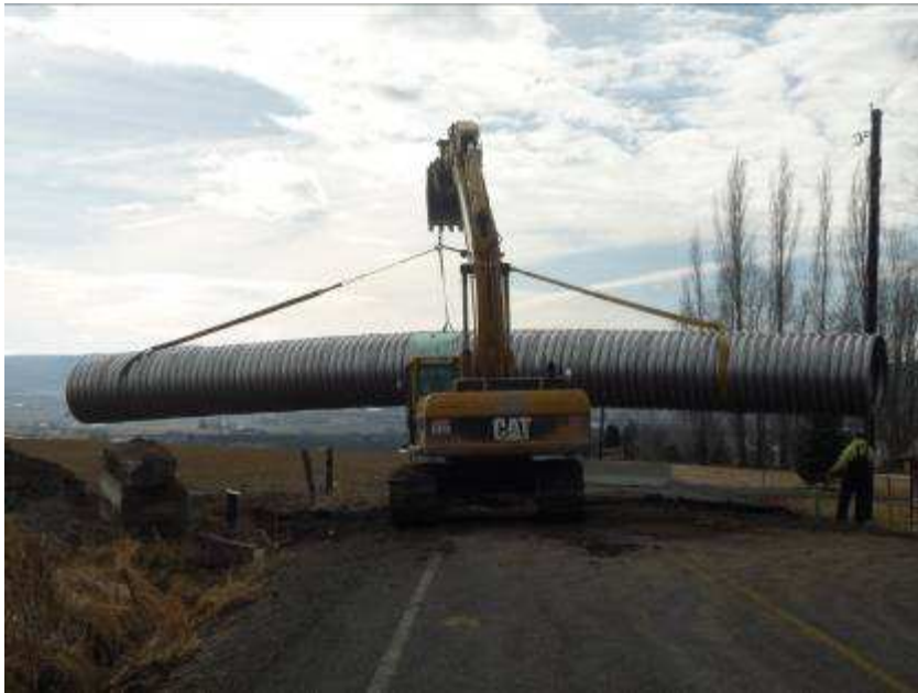
New Culvert on Site-Cleman Road Bridge
