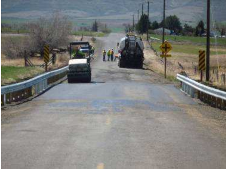
Paving on Badger Pocket Bridge
