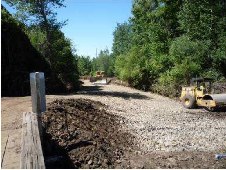
Construction of Bridge Approaches on Cooke Canyon Road
