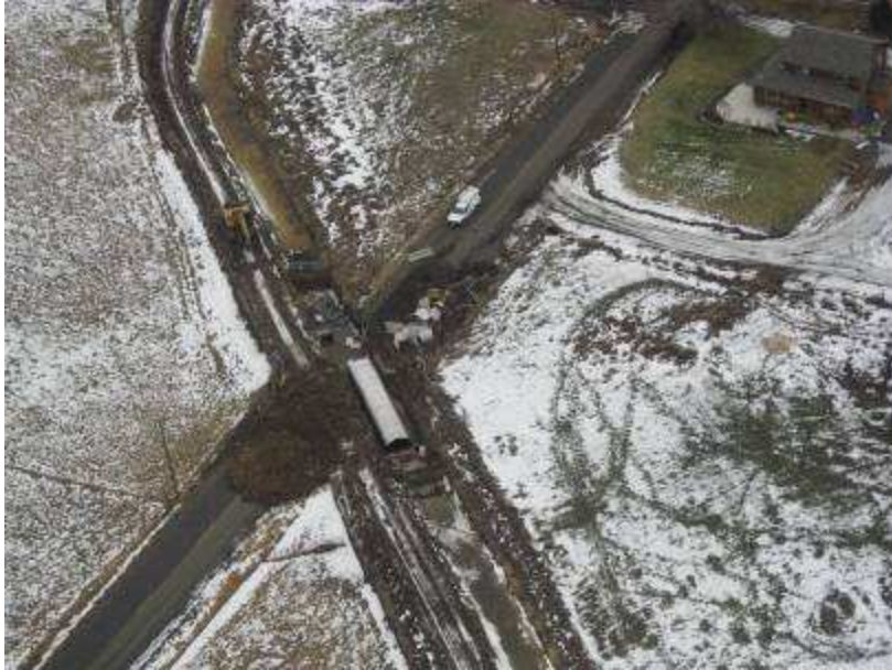
Aerial Shot of Construction Site –Carroll Road Bridge
