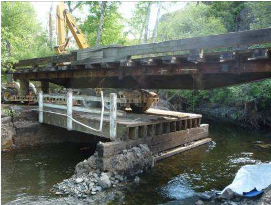
New Temporary Bridge Being Placed on Cooke Canyon Road
