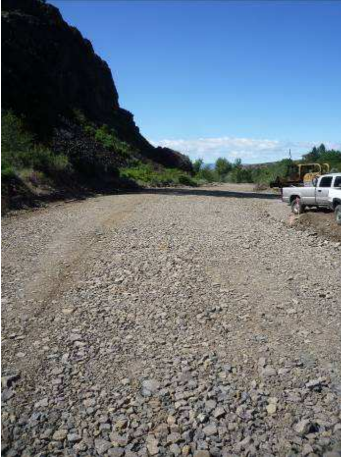
Repairs Underway on Cooke Canyon Road
