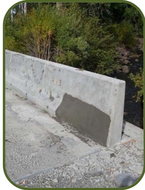
Finish Work for Traffic Barrier
