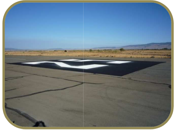
Project Completion- Application of Sealant & Paint Stripe of "25" Runway Numbers
