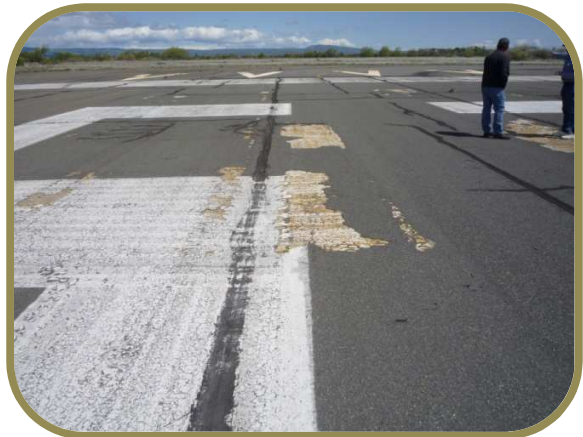
Example of the De-Lamination of the Old Chip Seal That Creates a Foreign Object Danger to Aircraft
