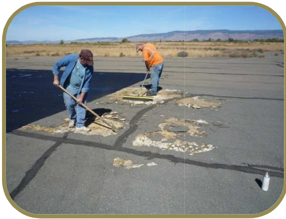
Removal of Old Loose Chip Seal Using Scrapers & High Pressure Air
