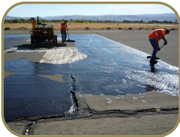
Project Completion- Application of Sealant to Project Area
